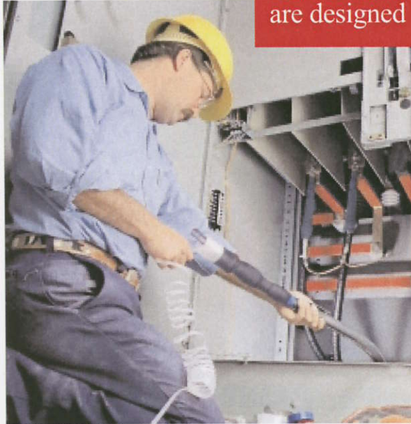
Cold Shrink QT-III Indoor Termination
