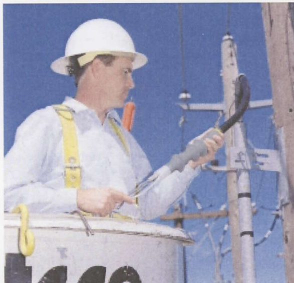
Cold Shrink QT-III Outdoor Termination
