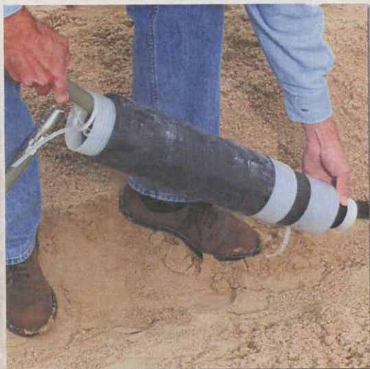
1. Prepare cable and position 3M™ Cold Shrink QS-III Splice components
